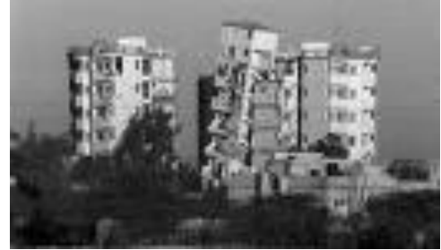
Fig.3. Damage to tall structures at Ahmedabad (India). The City of Ahmedabad is 320 km from epicenter.
