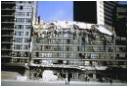
Fig.2 Failure of Hotel Continental in Mexico City. Site located at 410 km from epicenter.
