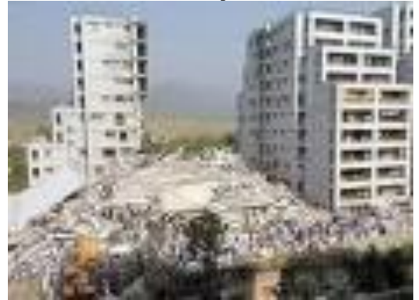
Fig. 4. Damage to tall building at Islamabad in Pakistan. The damage site located at a distance of 150 km from epicenter.
